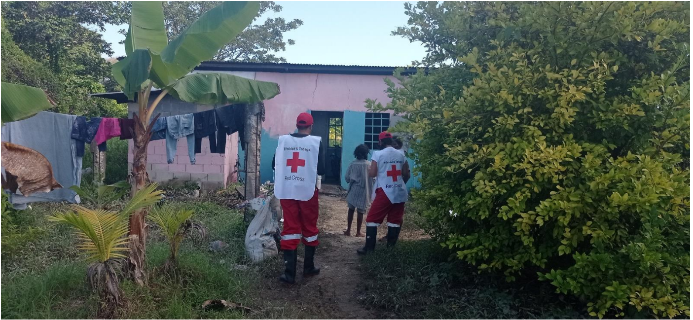
Figure 3: TTRCS Crisis Response Team conducting damage assessments at an affected home in the Mafeking area. 01Dec2022. Source: TTRCS
