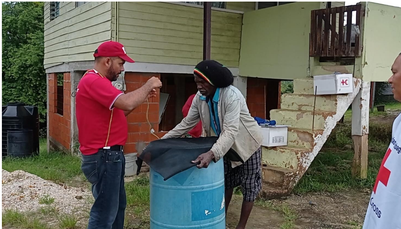
Figure 2: TTRCS Community Liaison Officer, Julio Pereira, teaches a Cotton Hill resident the proper technique of “drum-proofing” using mosquito netting and elastic cords to create a filter to prevent mosquitos from breeding in their drums, as well as keep foreign debris out, while still being able to collect the rain water from the guttering of the home. Credit, TTRCS August 2022.
